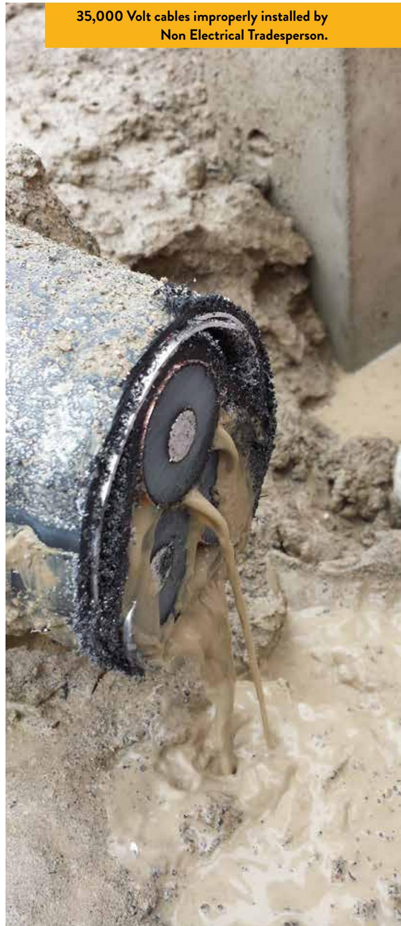
**35,000 Volt cables improperly installed by Non Electrical Tradesperson.**
